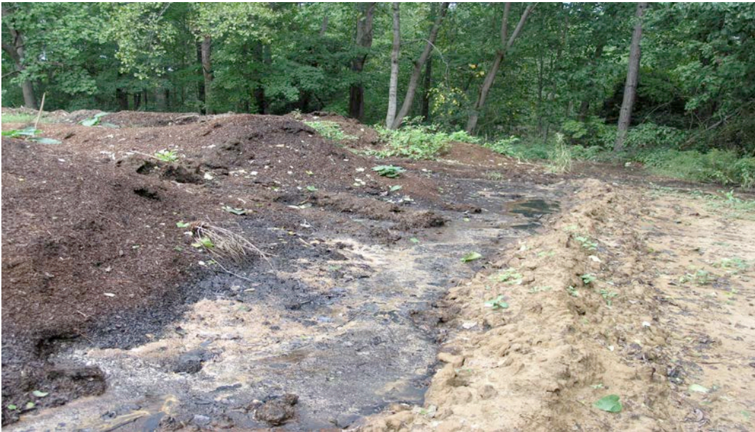
At the east end of the pile it is obvious how the “berm” merely funnels water into the ravine. The black water between the pile and the “berm” contained 170 ppb arsenic.
